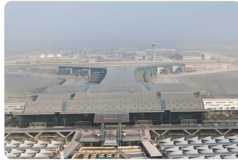
Roof of Doha Airport in Qatar. Picture courtesy of Hamad International Airport
