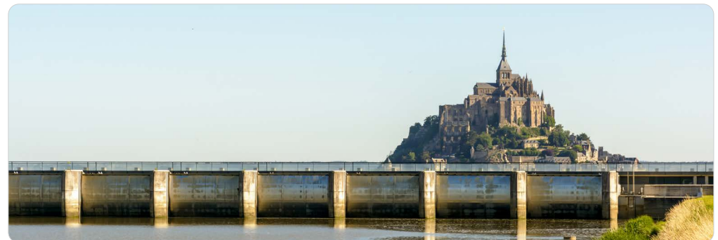
Sluice gates and Mont Saint Michel, France.
