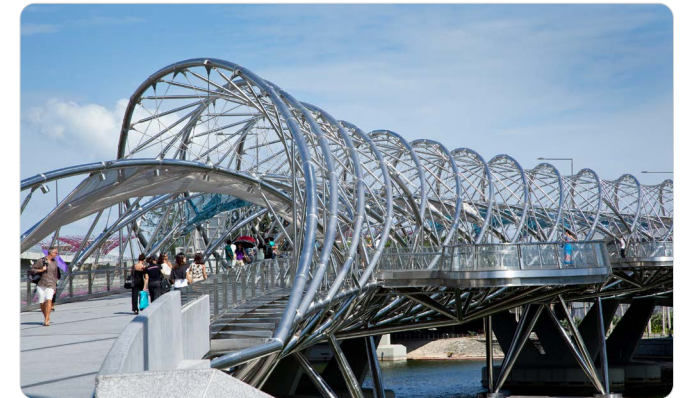
Helix Bridge in Singapore Picture courtesy of Christopher Fredrick Jones
