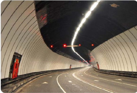
Lining of the Queensway tunnel in Liverpool Picture courtesy of Ancon Ltd
