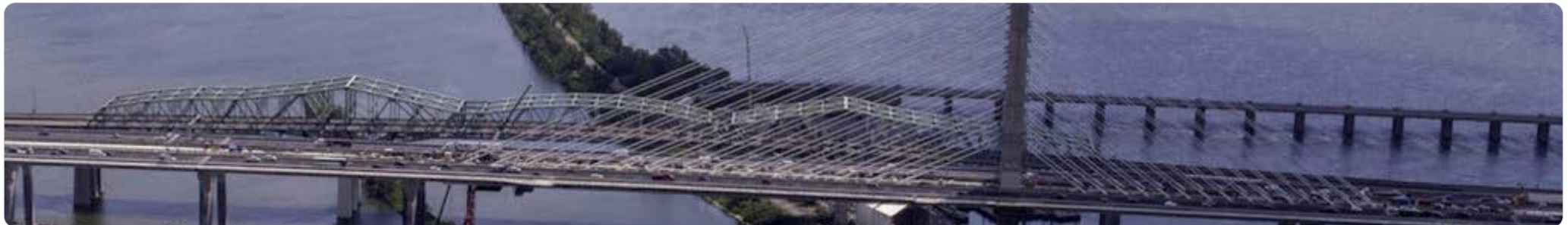
Champlain Bridge in Montreal, Canada. Picture courtesy of Infrastructure Canada
