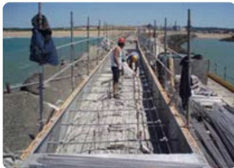
Breakwater in Bayonne, France Picture courtesy of Ugitech S.A.
