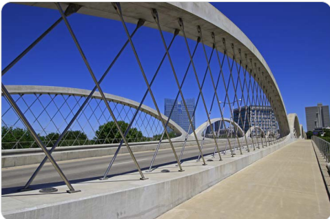
Fort Worth bridge in Texas
