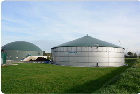
Duplex stainless biogas tank Picture courtesy of Börger GmbH
