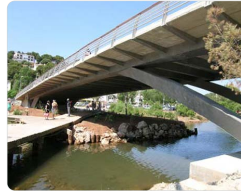
Cala Galdana bridge in Menorca Picture courtesy of Pedelta
