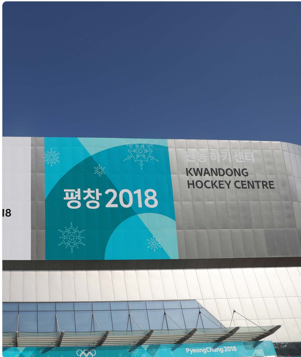
Detail of the Kwandong Ice Hockey Center in Korea, clad in lean duplex 329LD
